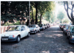
Intimate tree-lined streets in yorkstone setts and boundary treatment consisting of brick walls stone copings and cast iron railings are characteristic of this area
