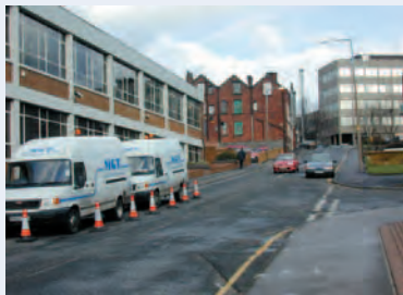
Typical post war industrial development south of Burley Road in need of enhancement (above)
