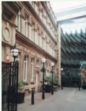
Conversion and new build make The Bourse an apt and exciting office development
