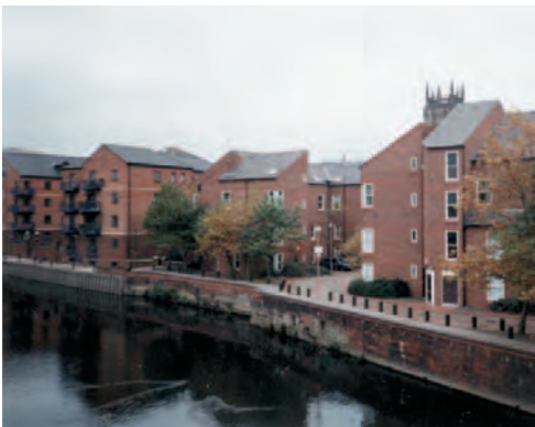
Enhancing riverside housing, The Chandlers, Call Lane (below)
