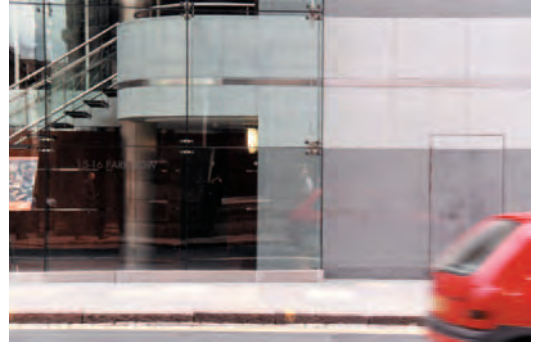
Concealed / under emphasised fire exit door at No. 15/16 Park Row (right side)
