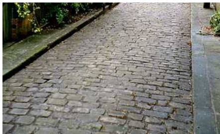
Stone walls are also an important feature and areas of stone sett paving, though few in number, provide texture and contrast at ground level (left, Back Heatherfield Terrace)
