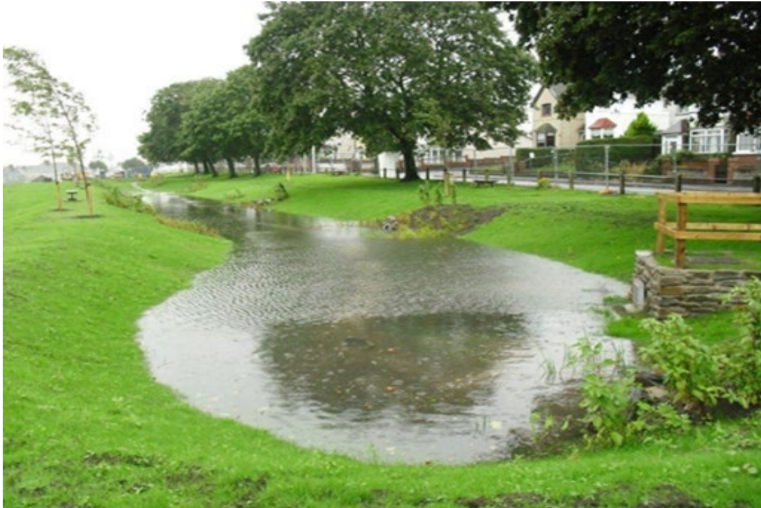
Photo: An example of the use of sustainable drainage
