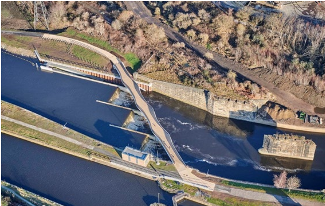
Photo: Construction of the Leeds Flood Alleviation Scheme
