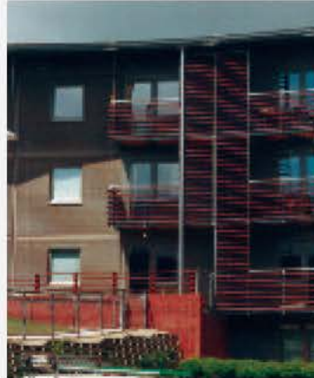
RECENT LOW RISE BLOCK OF AFFORDABLE FLATS TO RENT Attractive, award-winning design
