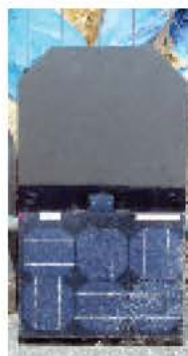
SOLAR SLATES Electricity generated for the householder by use of solar slates on the roof in this Housing Association scheme
