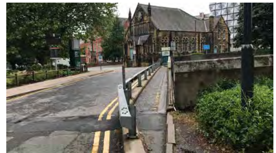
↑ Willow Terrace Road Crossing over Leeds Inner Ring Road
