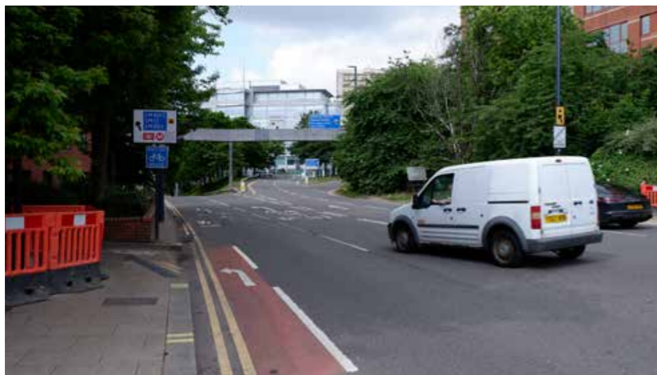
↑ Confusing and unsafe cycle and pedestrian environment at Westgate
