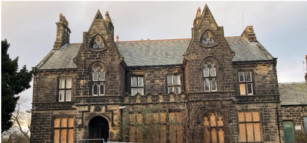
Micklefield House, awaiting conversion
