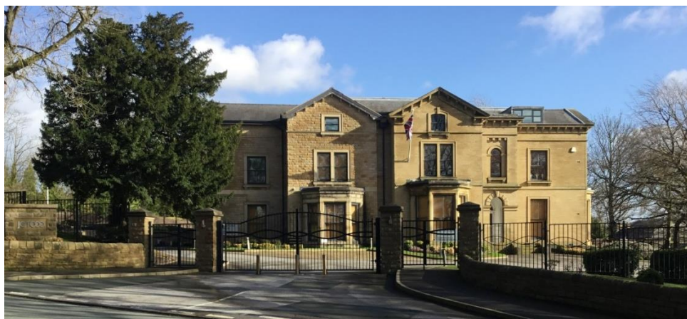
Headquarters of JCT600 Group, Apperley Lane
