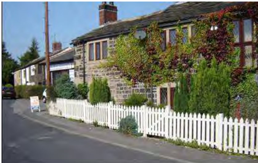
Listed cottages on Low Moor Side. The stone window surrounds are a characteristic feature set in the coursed gritstone, but the facades tend to be obscured by the Virginia creeper.
