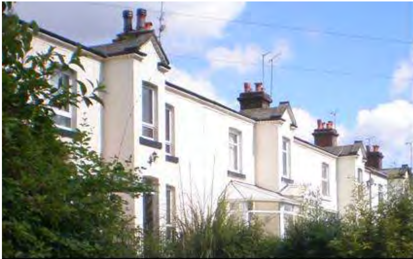
Croft Terrace. 19 th century housing for under-managers at the Famley iron Works, given additional "presence" by the pedimented two storey porches
