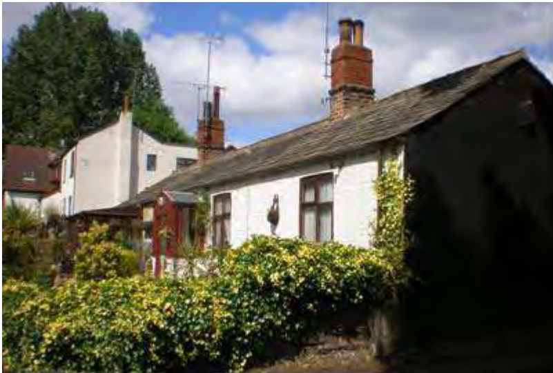
Croft Cottage. White painted brick under a slate roof. A contrast in scale with adjoining properties adding to the variety on the Coach Road.
