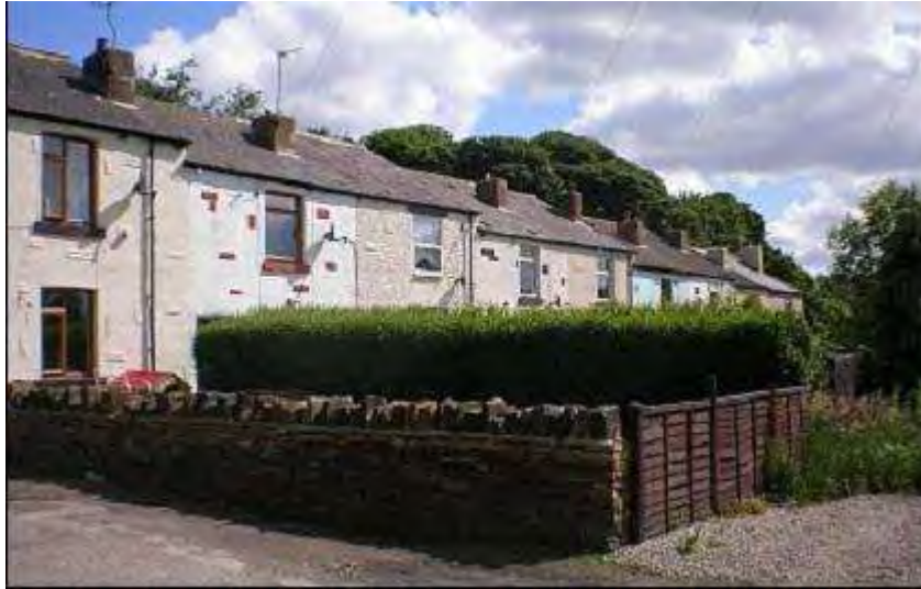
Forge Row. Terrace constructed for workers at Farnley Ironworks. Some houses have had cosmetic treatment to their façades which detracts from the overall character of the terrace
