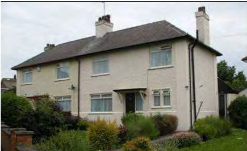
Wolley Avenue. 1930s estate for workers at Farnley Iron Company, unspoilt by dormers and extensions
