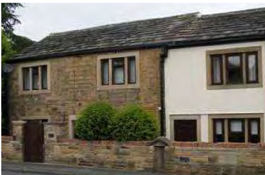
Low Moor Side. Vernacular cottages with typical stone window surrounds
