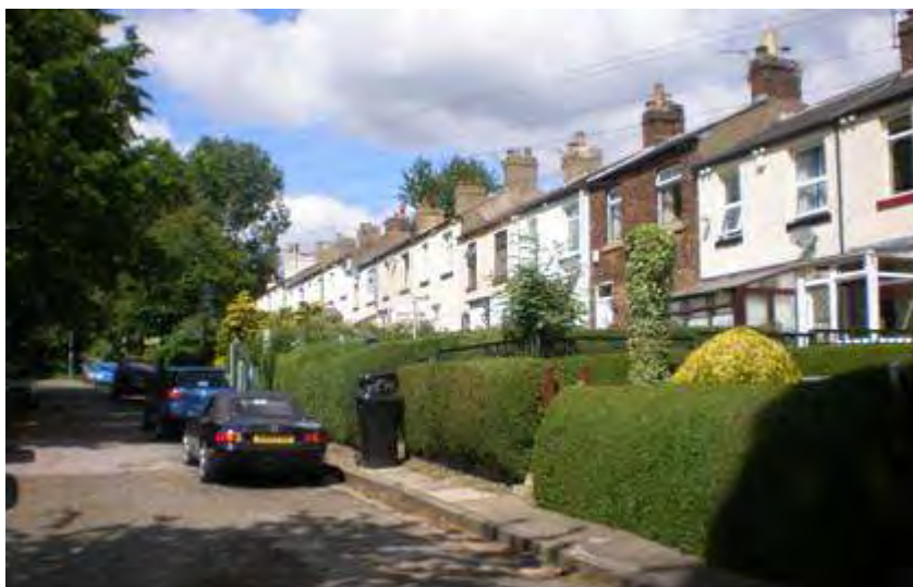
Playground. Garden hedges and chimneys are a positive feature of this terrace. The original brick has been exposed on one house, affecting the unity of the terrace.
