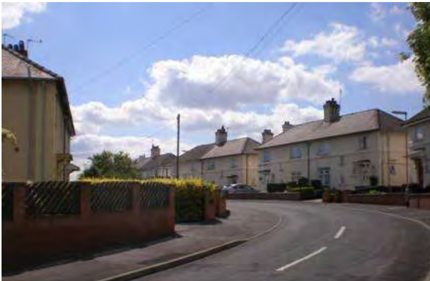
Wolley Avenue. Wide-fronted rendered houses with hipped roofs, arranged in a sweeping curve. Most have remained unaltered, maintaining the integrity of the original design.
