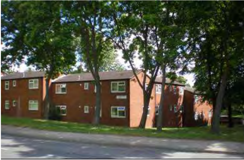
Gainsborough Place, viewed from Lawns Lane. The trees make this development more attractive than it would be without them.
