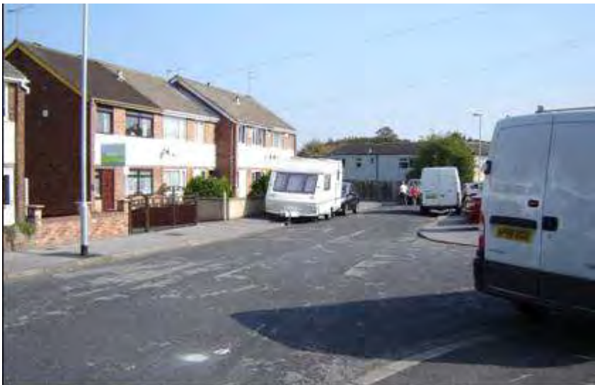
Wolley Drive. The original design included grouped garages, leading to problems with parking.
