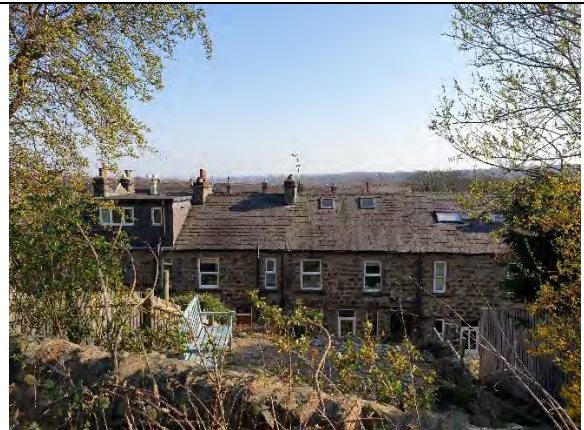
Figure 14: SE from Wood Lane.
