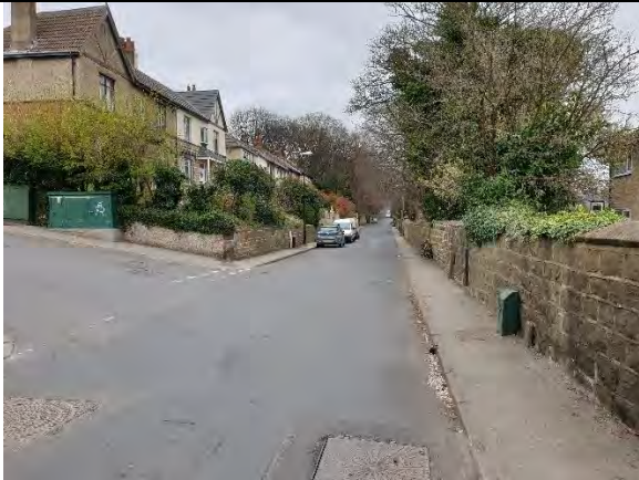
Figure 27: NE from Newlathes Road into Newlay Lane.
