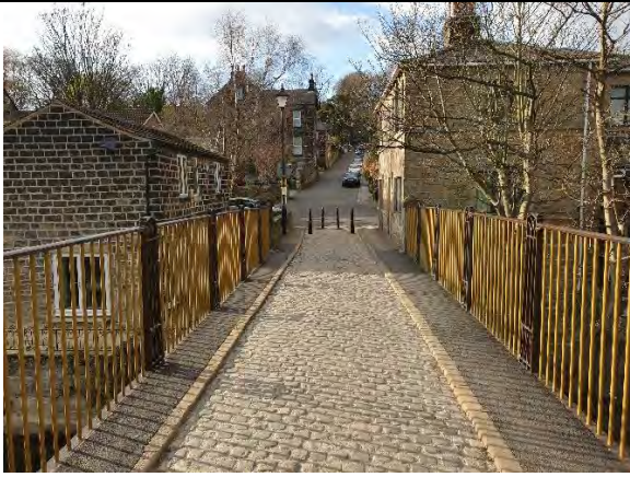
Figure 1: NW from Newlay Bridge to Newlay Lane.
