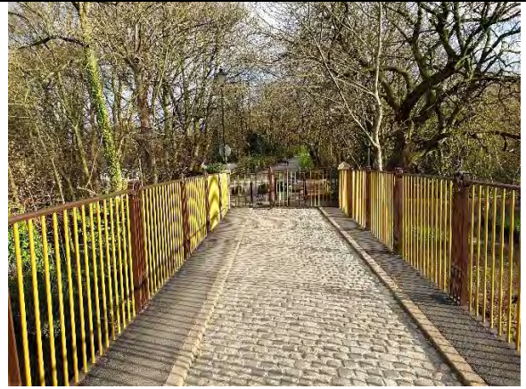
Figure 2: SE from Newlay Bridge to Pollard Lane.
