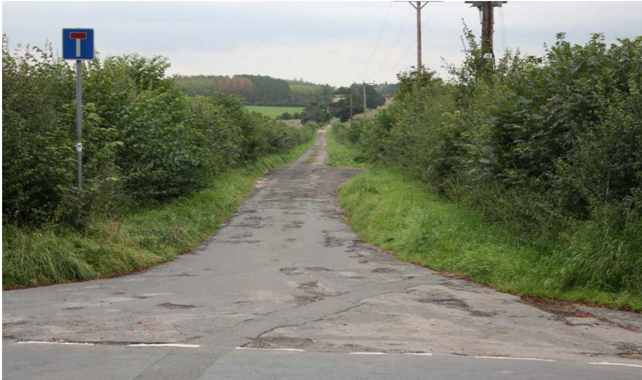
LR1. From Aberford Road south east down Headley Lane
